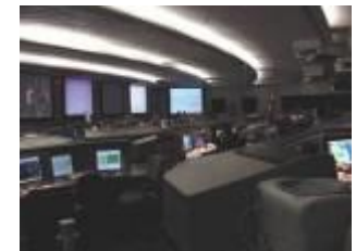
2 Operational Control Centers
