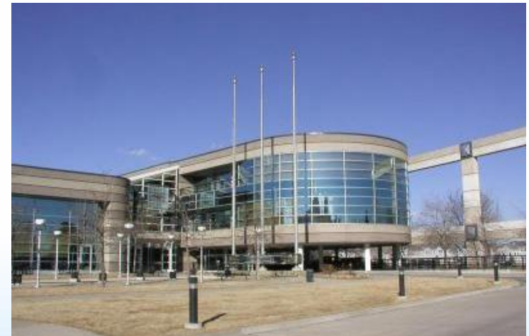
UCAR Center Green Facility
