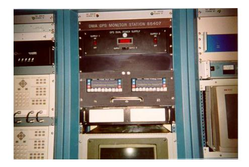
The NGA GPS Tracking Station at USNO uses a frequency standard tied to UTC(USNO)
